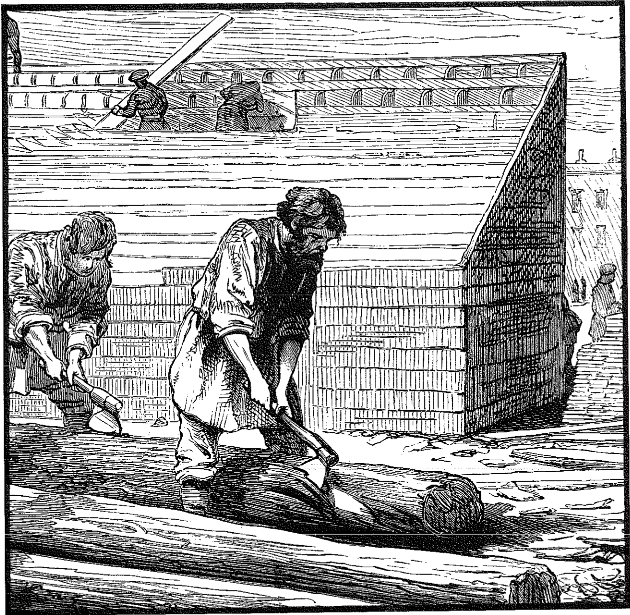
SQUARING OFF LOGS WITH A BROAD AXE THE BETTER FOR STACKING AND KNITTING THEM SNUG
